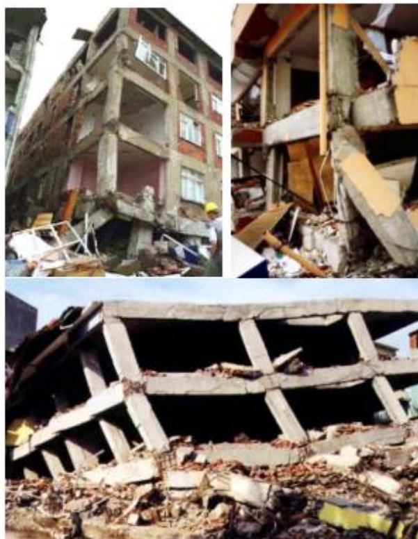
Figure 1.4 Collapse of the reinforced concrete building; a) Turkey, Duzce earthquake, 1999; b) Sarpole-Zahab earthquake, Iran 2017 [10][11].
