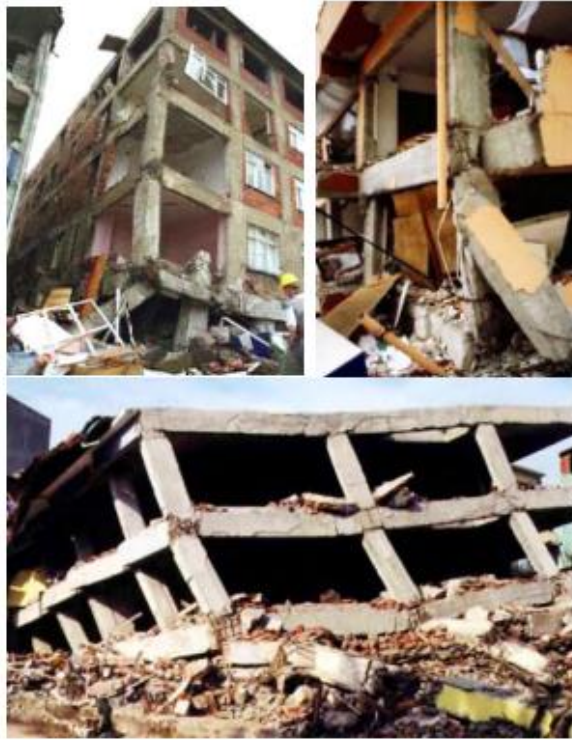
Figure 1.3 Buildings collapse due to failure of beam-column joints, Izmit, Turkey, Earthquake in 1999 [9], [9]. (a) (b) (c)
