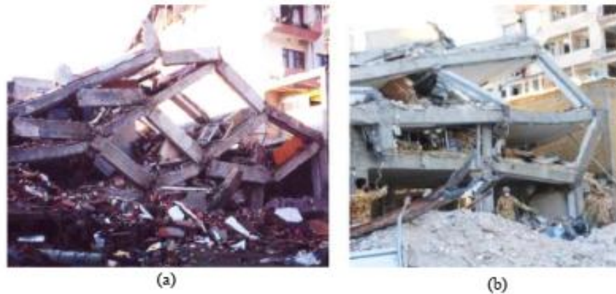
Figure 1.5 Damage to partial damage of reinforced concrete building due to beamcolumn failure in Chi-Chi, Taiwan, earthquake, 1999 [12]
