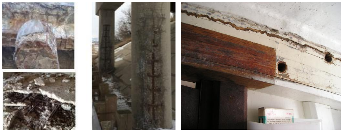
(A) Corrosion of columns
